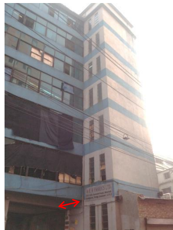
Cantilever – North Façade Approx. 0.8m
