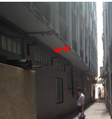
Cantilever – South Façade Approx. 1.6m
