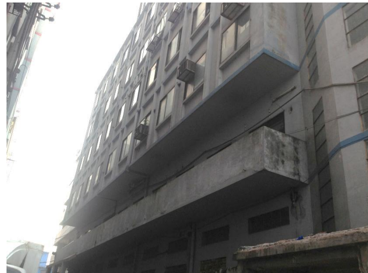
Cantilever – East Façade Approx. 1.0m
