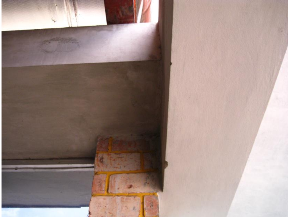
Front side: Movement joint should be here
