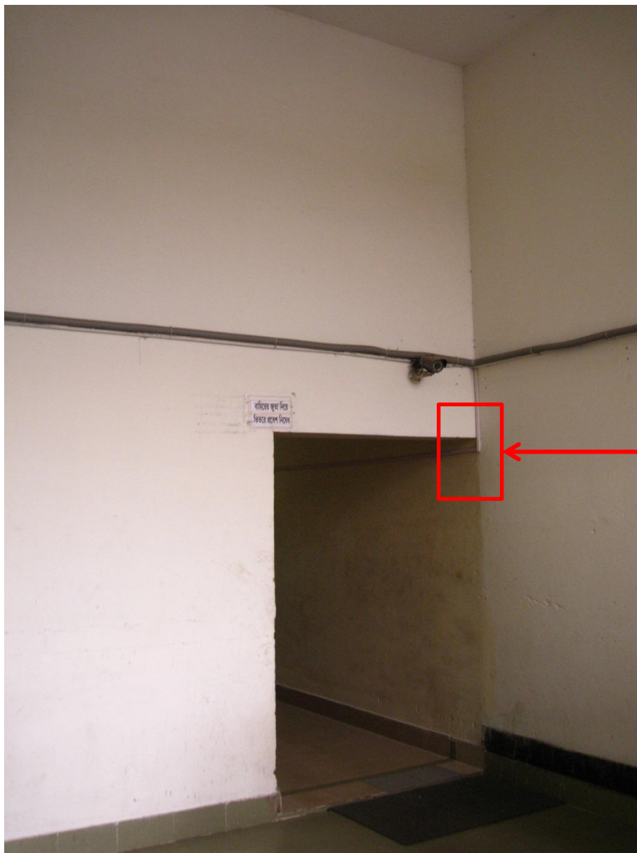
Elevation of Lintel
