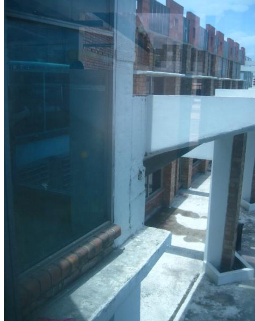
Back side: Movement joint in façade
