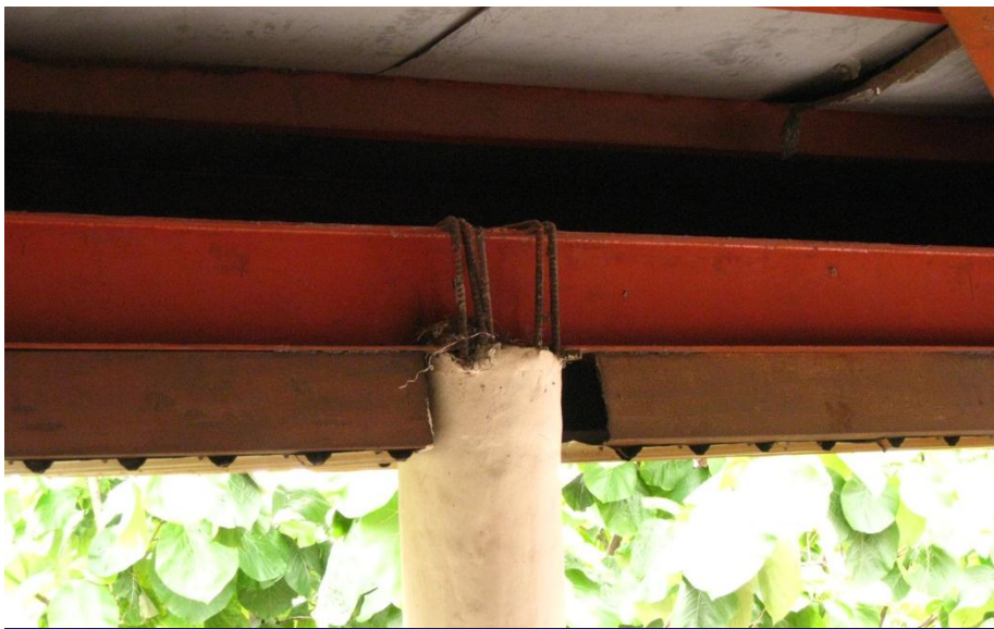
Building 1 – RC column to steel beam connection
