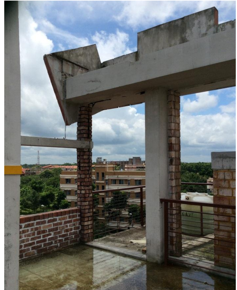
Inadequate supports
