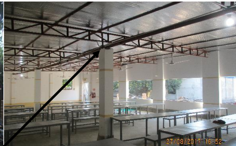
Typical truss frame which supported by reinforcement column
