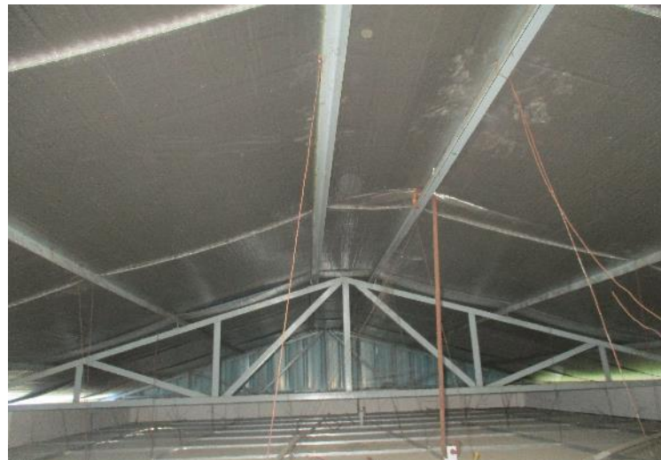
Typical internal truss
