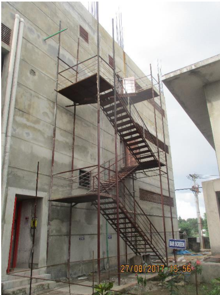
South side Steel stair
