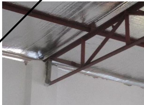
Corner joint between RC column and truss
