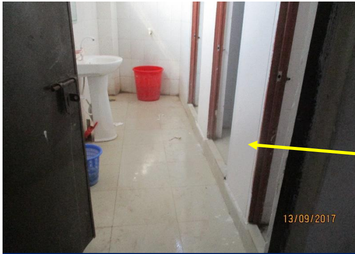
Toilet partition walls
