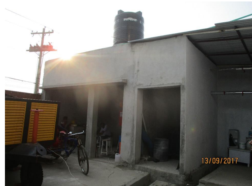
Utility Building (Boiler)
