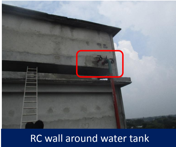
R.C.C water tank
