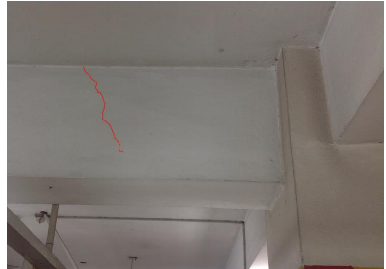
Crack in beam – u/side 8 th floor
