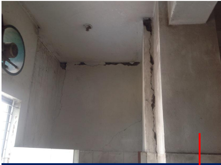
Cracking to 8 th Floor Washroom
