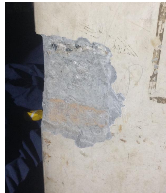
Tested Ground Floor Column
