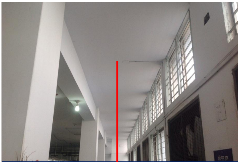
2m cantilevering slab (no down-stand beams)
