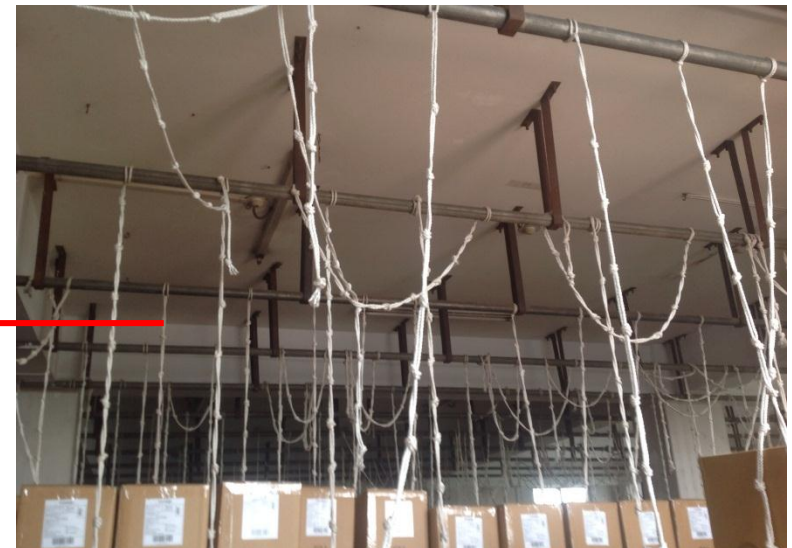
1 st Floor Storage Area – Hanging Point Loading
