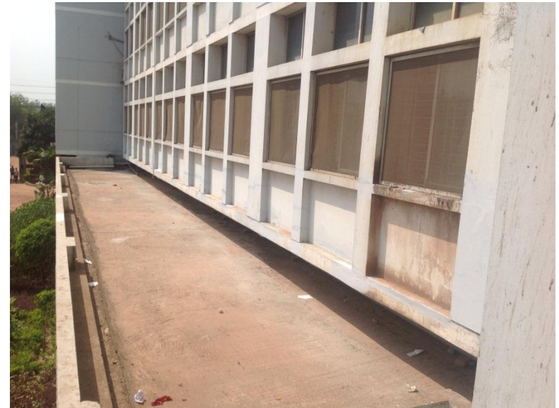
View of Façade at 1 st Floor
