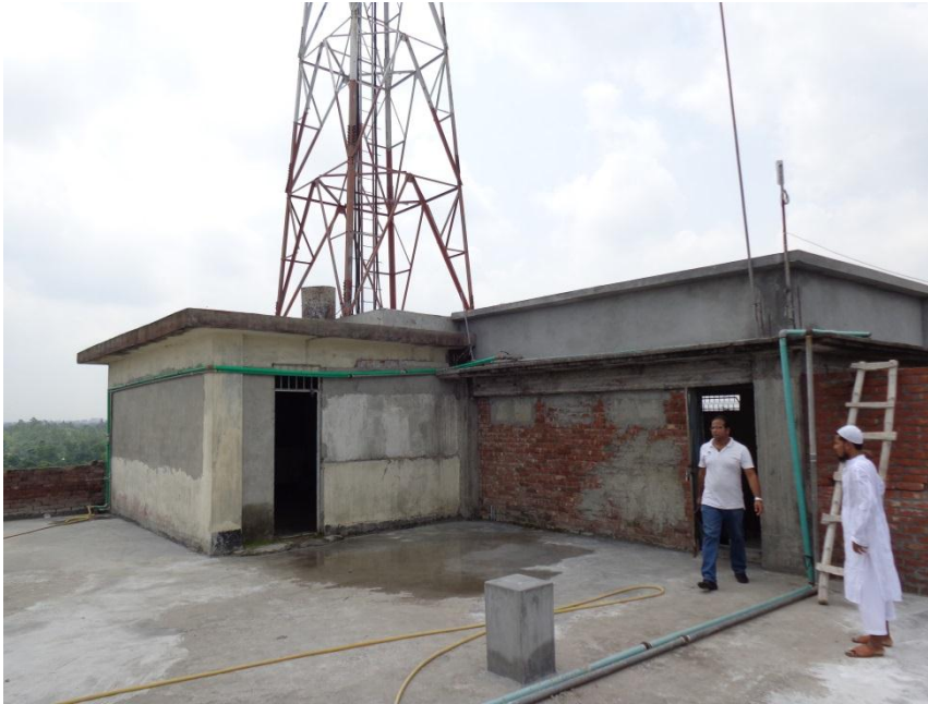
Critical Column at Original Building
