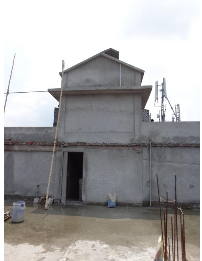
Critical Column at Extension Portion
