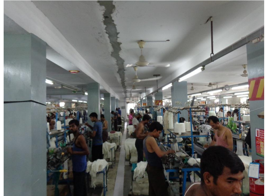
Plaster Repair along Joint
