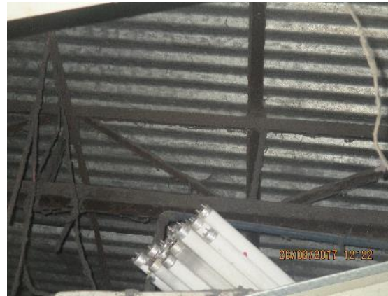
Steel truss frame
