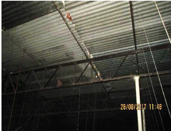
Steel truss frame of Cutting Shed
