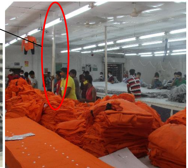
Steel pipe column
