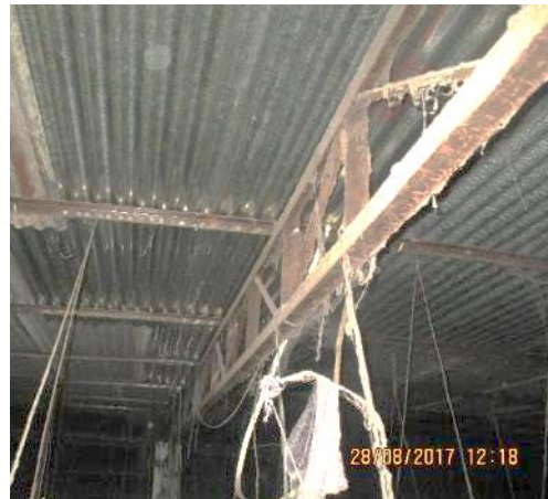
Steel roof truss
