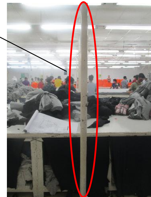
Steel pipe column
