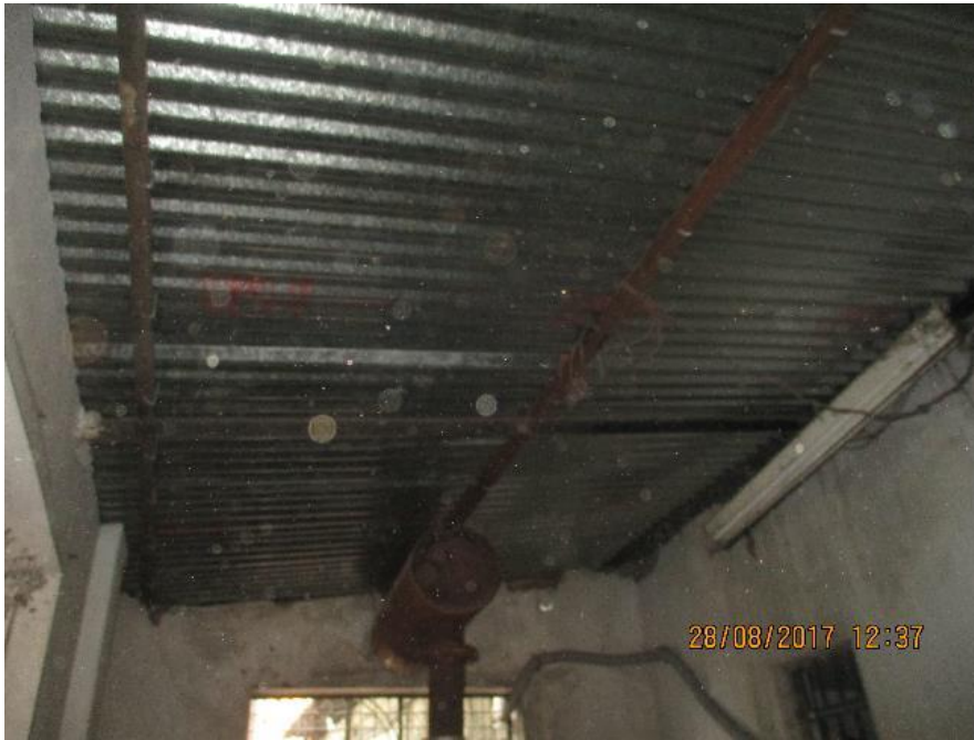
Roof system of the Generator shed
