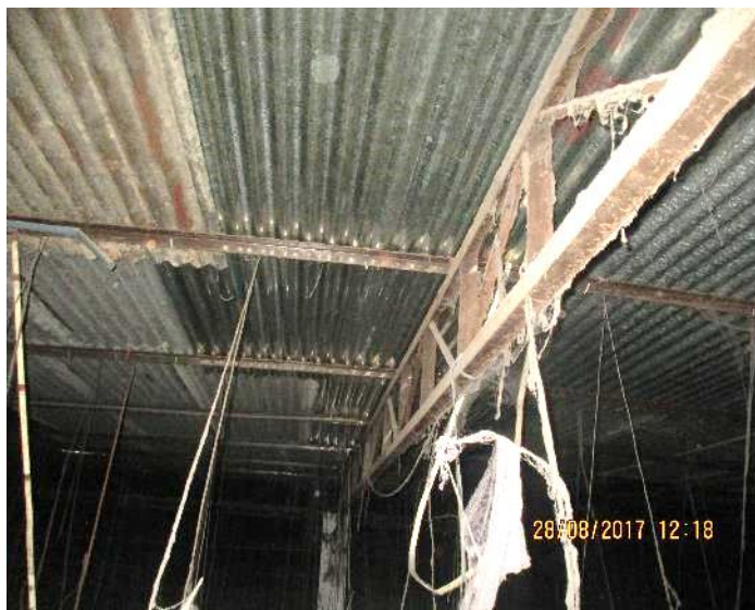
Steel truss frame of Sewing Shed
