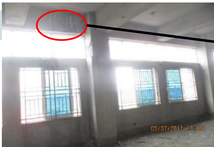
Dampness was found on beam slab joint on exterior side
