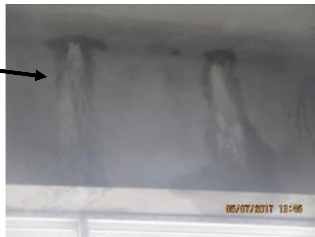
Dampness was found on beam slab joint on exterior side
