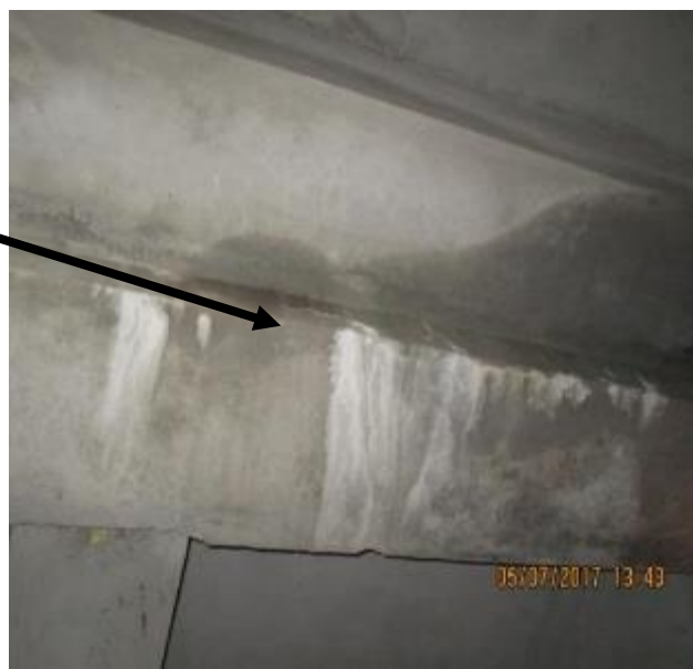
Excessive dampness was found on movement joint of toilet area(6 th floor)
