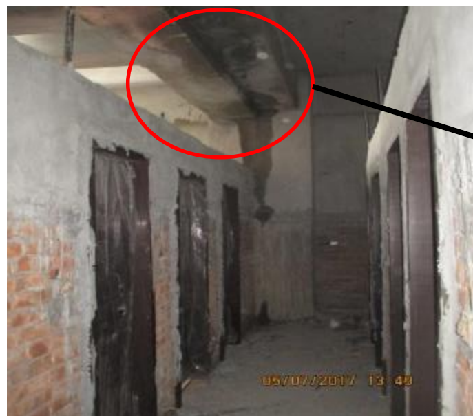
Excessive dampness was found on movement joint of toilet area(6 th floor)
