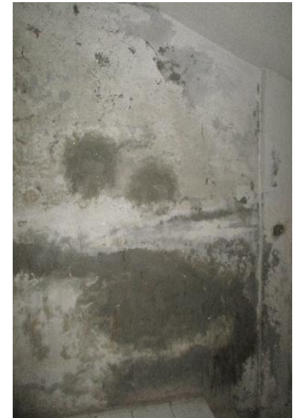
Dampness observed on stair portion
