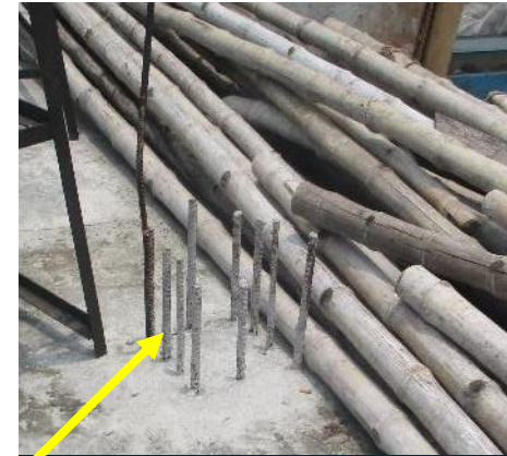
C1: 2- 16mm+5-20mm+2- 16mm on roof
