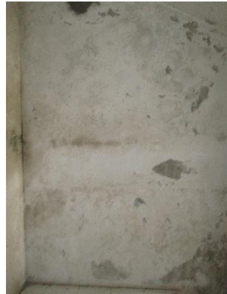
Dampness observed on stair portion
