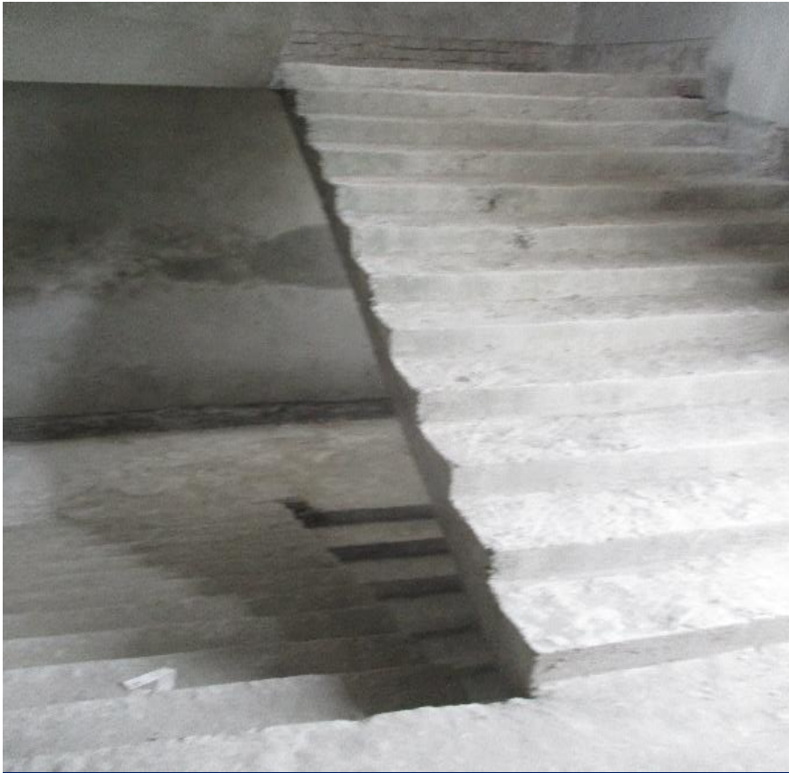
Stair- 01 portion(3 rd floor to roof)
