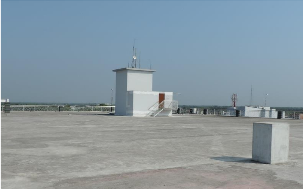
Water tank adjacent to lift room. Partially supported by lift core and partially supported on roof deck
