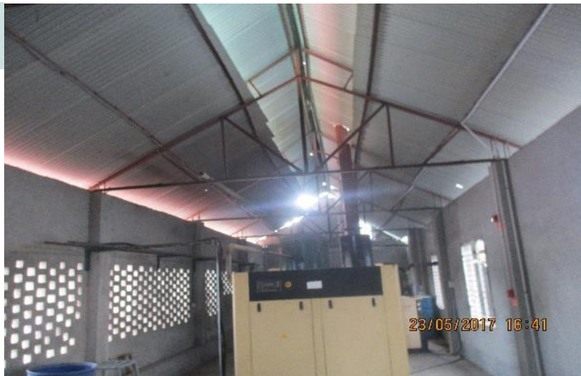
1 st floor roof shed of generator building
