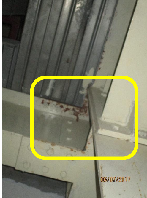
Corrosion at beam-column joint
