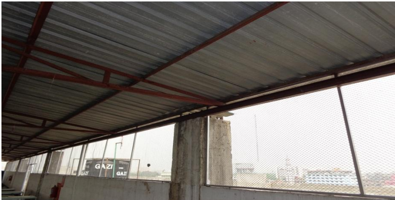
Roof made of structural steel.
