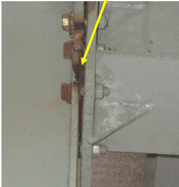
Tear on column-rafter joint
