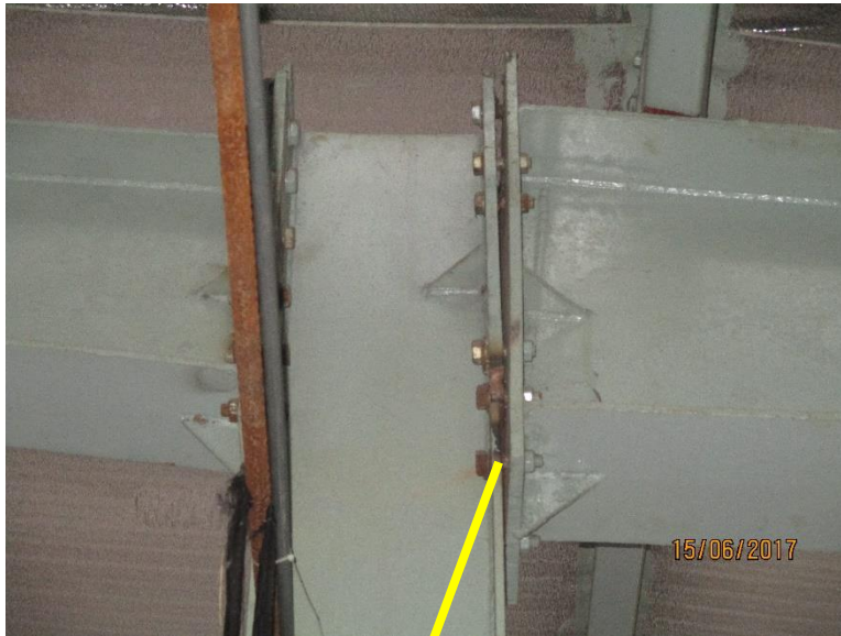
Tear on column-rafter joint
