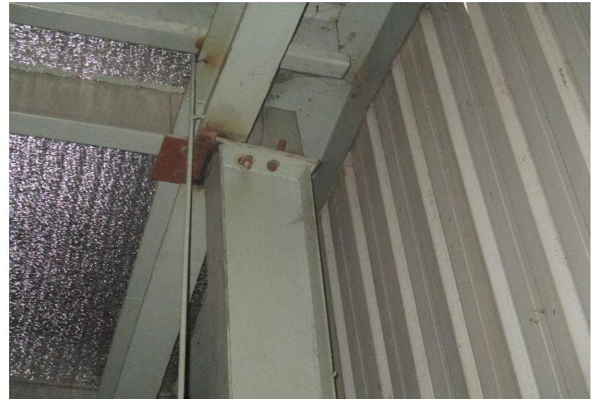
Additional steel plate added to support rafter
