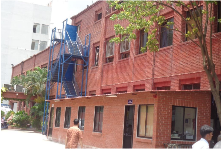
Main 3-storey building & adjacent staircase
