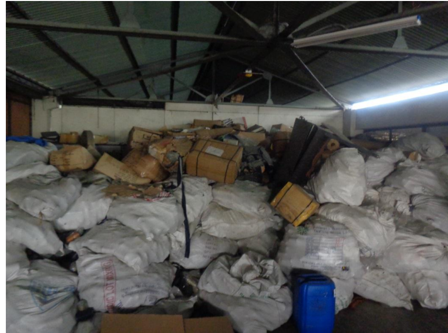
Storage Loading on 2 nd floor
