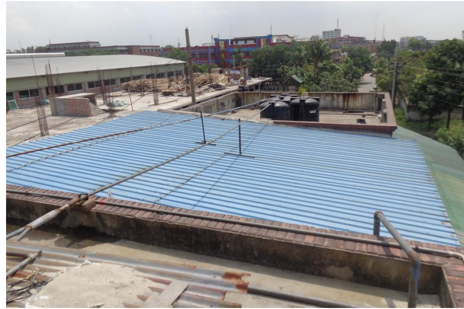
2-storey concrete extension
