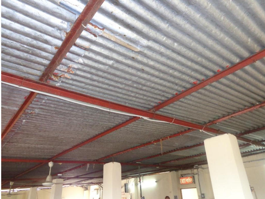
Steel roof on roof slab
