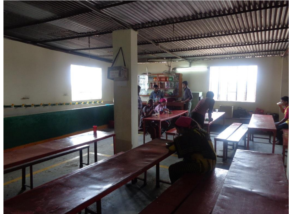
canteen & steel roof
