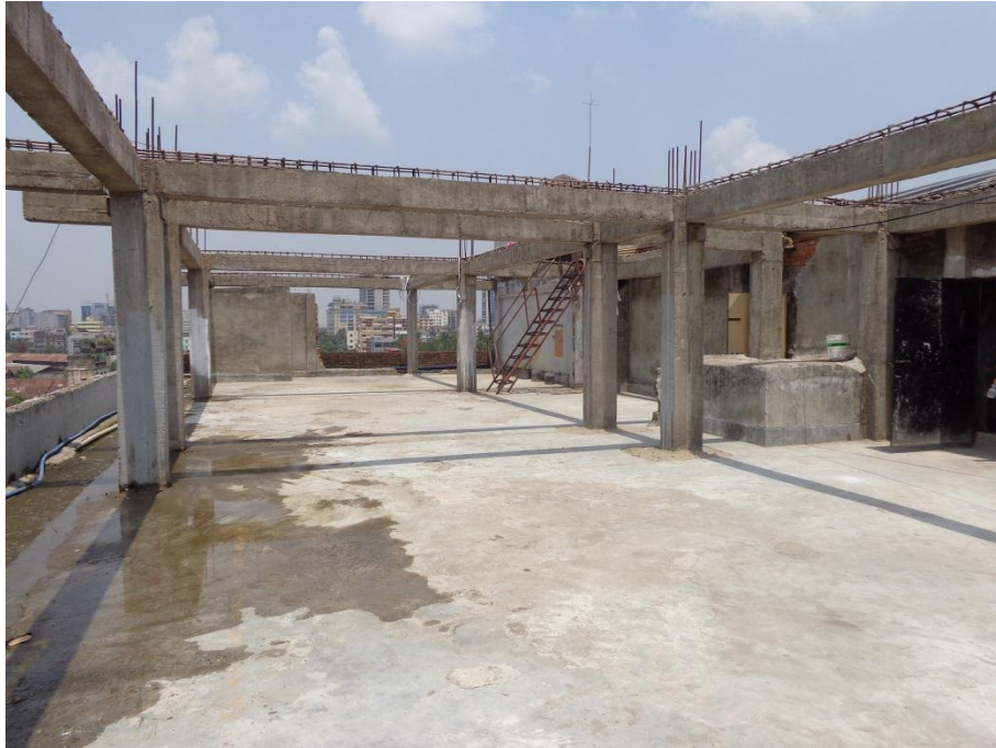
5 th floor roof slab
