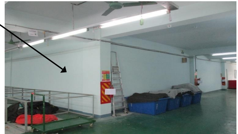
Full height brick walls on 1 st floor
