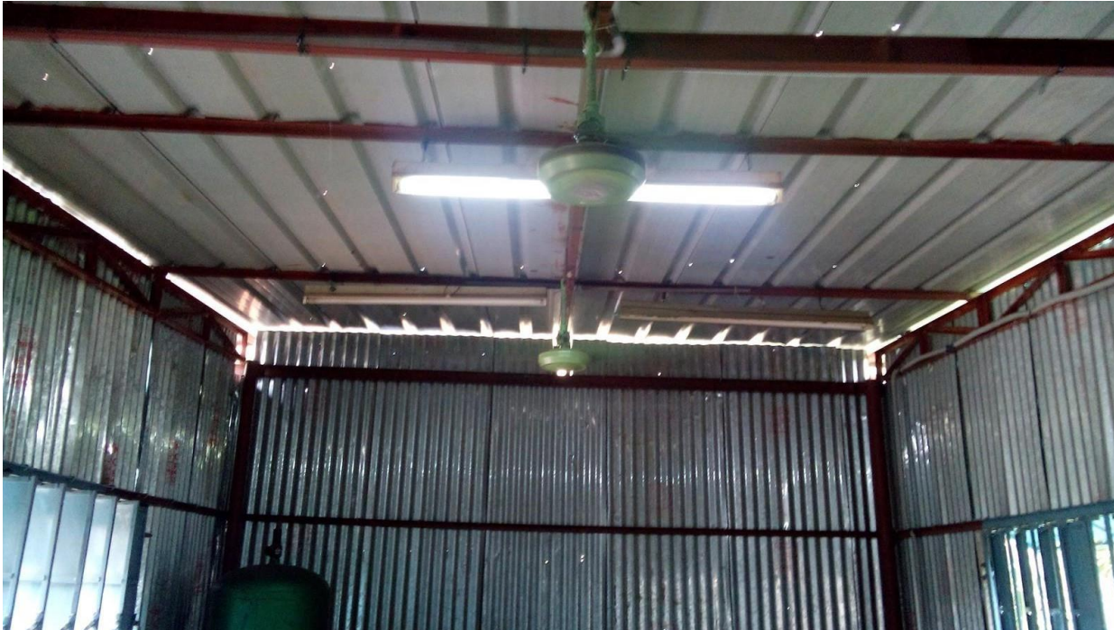
Lightweight steel truss supported roof cladding
