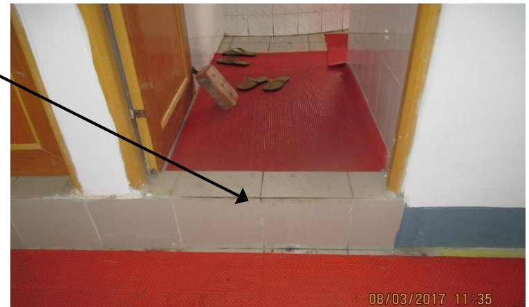
Additional toilets with 200mm ~ 350mm floor built up on 2 nd & 3 rd floor
