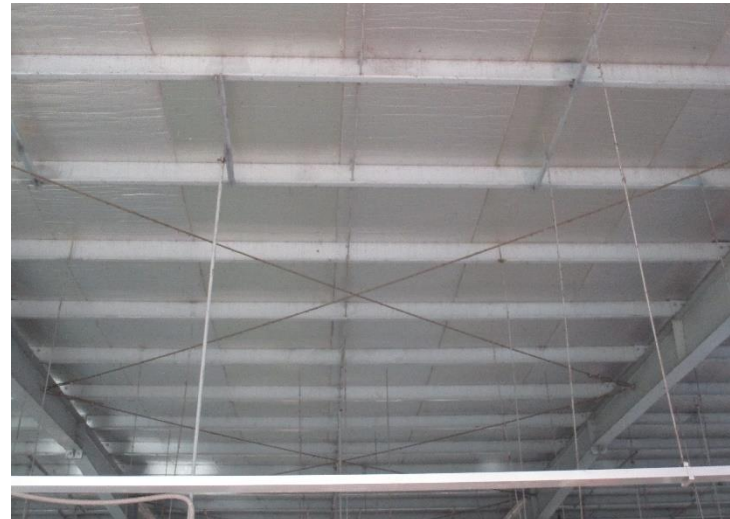
Roof Bracing
