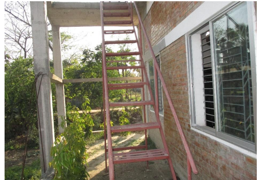
External steel stair at Generator & Sub-station
