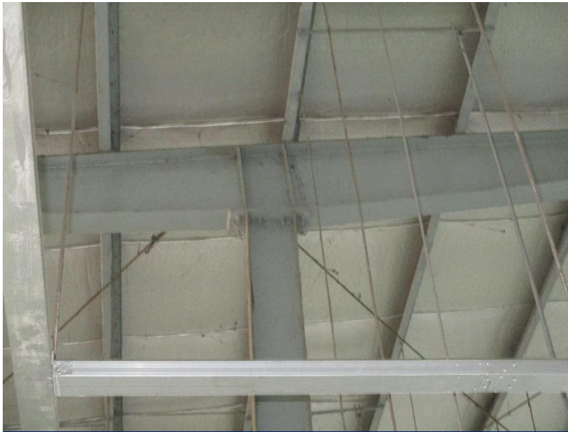
Beam column connection
