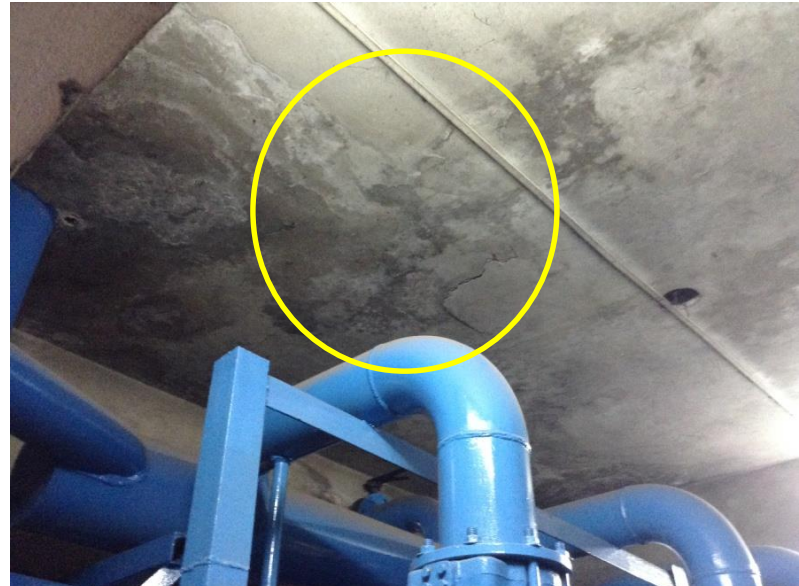
Few hairline cracks were observed on the ceiling slab
