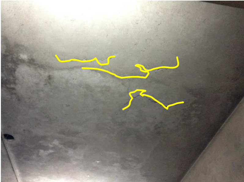
Few hairline cracks were observed on the ceiling slab
