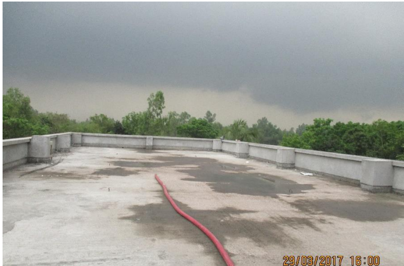
Utility building roof
