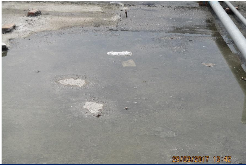
Water ponding on main factory building roof
