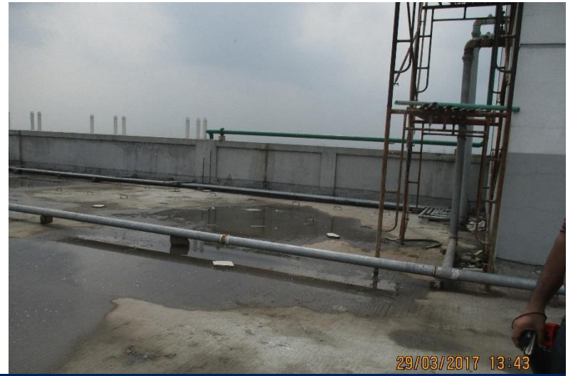
Water ponding on main factory building roof
