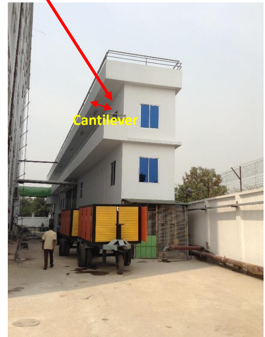
1.22m of Cantilever slab located front side of the building
