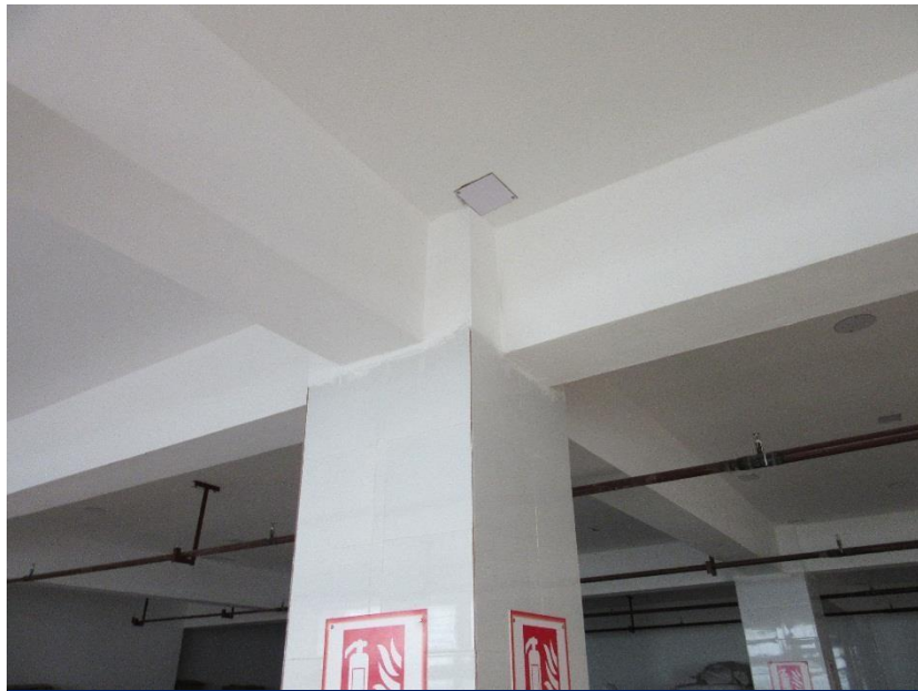
Typical Column Beam frame structure
