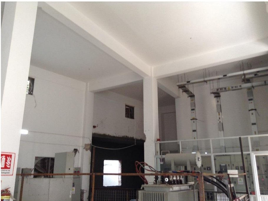
Typical Column Beam frame structure
