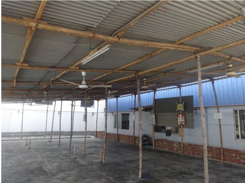
Structural condition of temporary buildings
