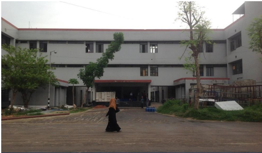
Front elevation of link bridge connected to Building 1
