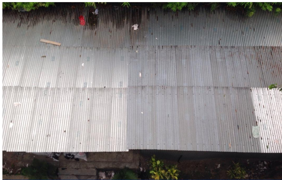
Building 2 – Lightweight structure at Ground level
