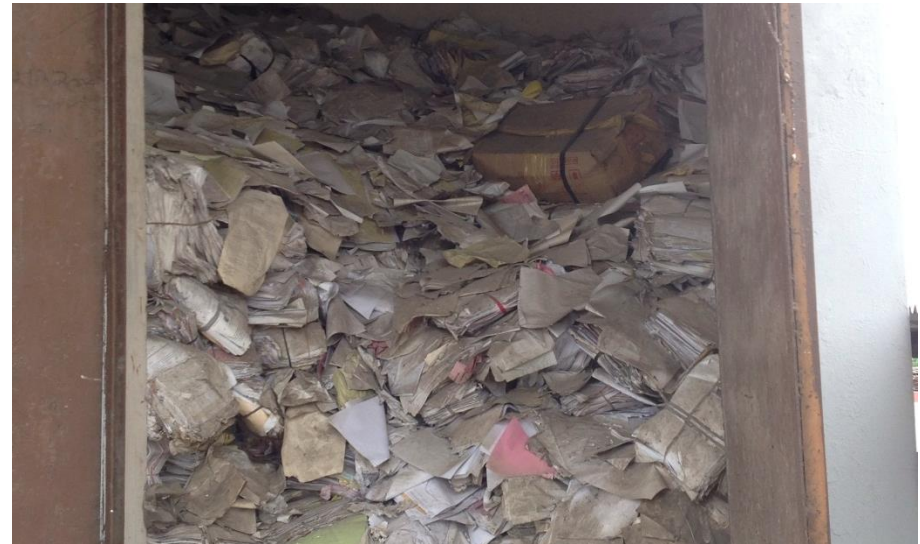
Building 1 - Storage room above lift-core at Roof level
