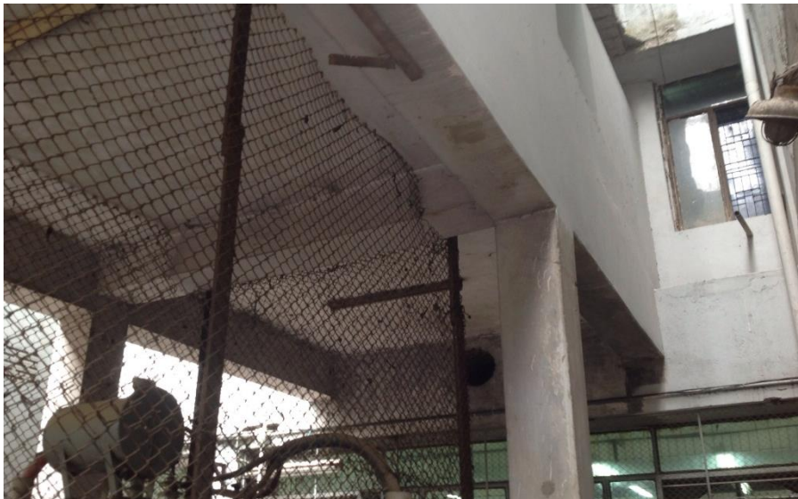
View of link bridge connection with Building 2
