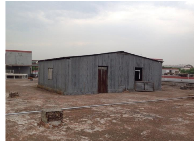
Building 1 – Lightweight Structure at Roof level
