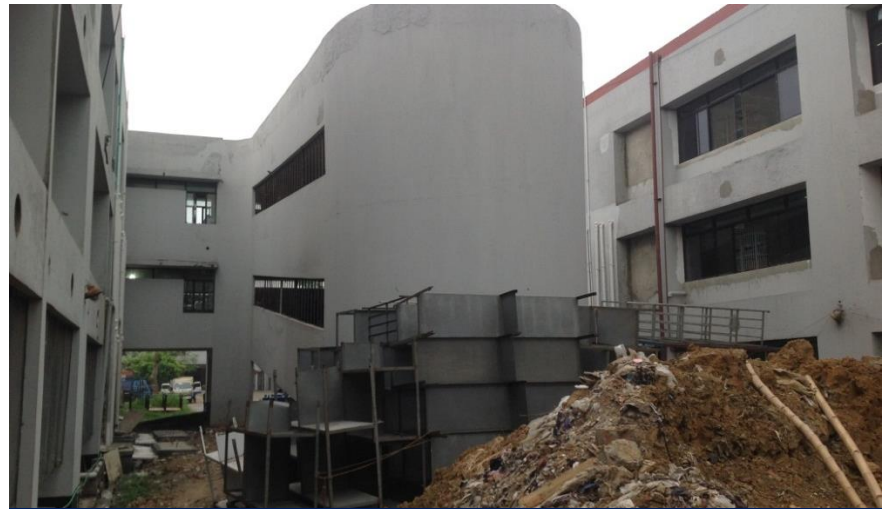
Back elevation of ramp and link bridge to Building 1
