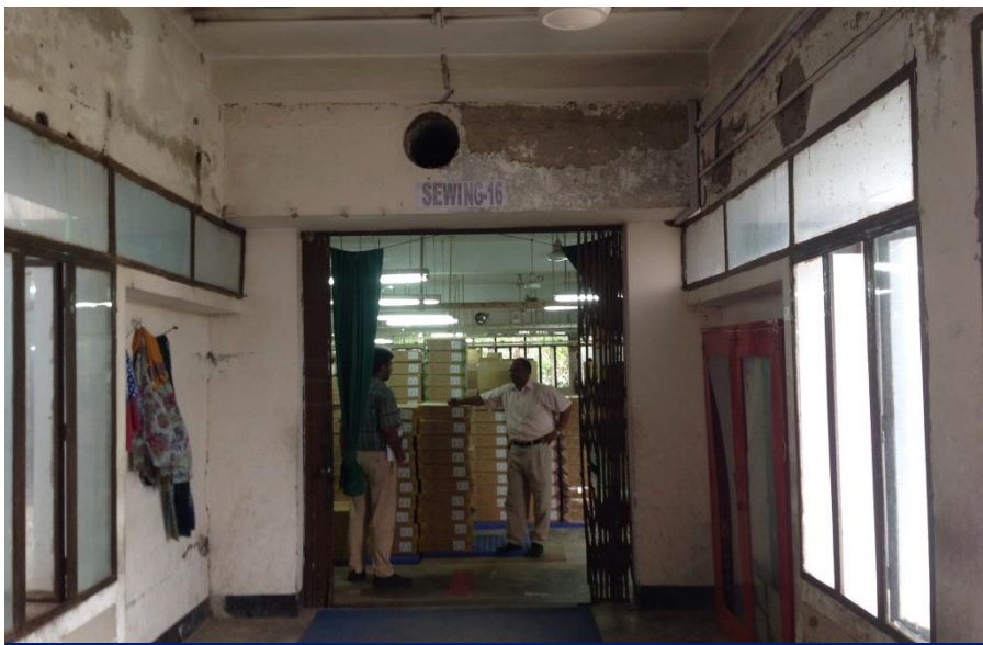
View from link bridge at connection with Building 1
