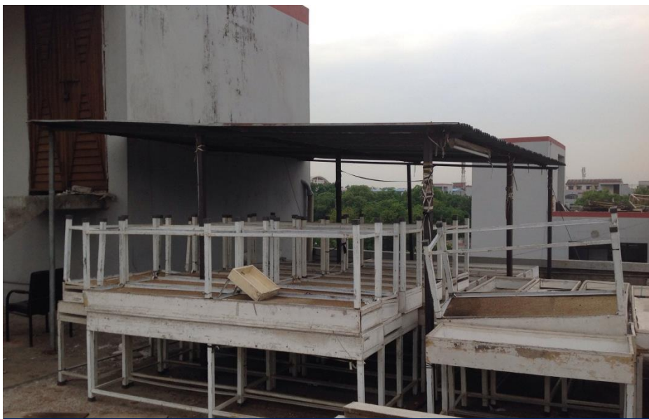
Building 1 – Lightweight structure at Roof level
