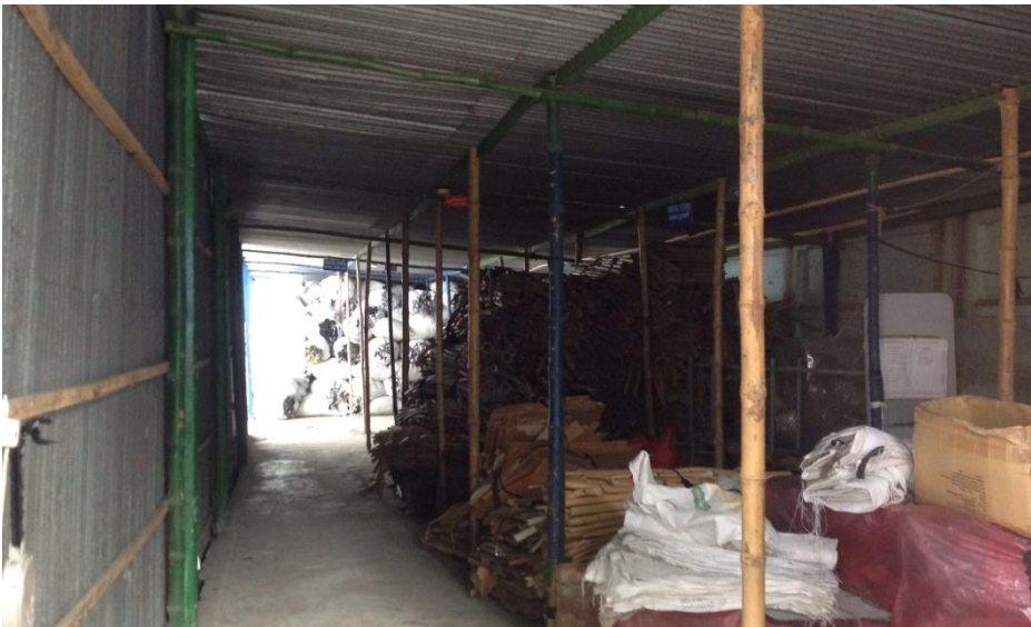
Building 2 – Lightweight structure at Ground level
