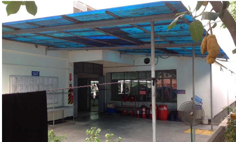
Building 2 – Lightweight structure at Ground level
