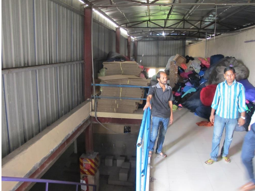
Steel Structure Bridges movement joint at roof level.
