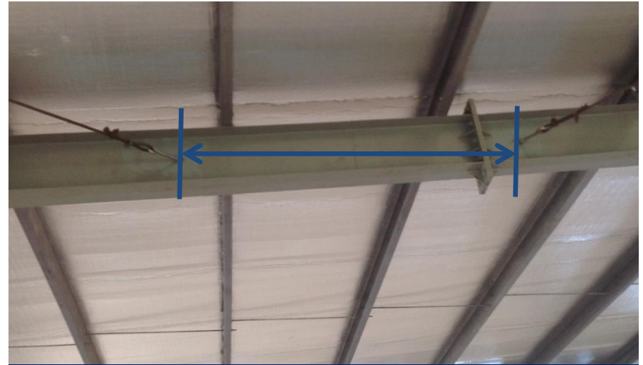
Significant eccentricity to plan bracings
