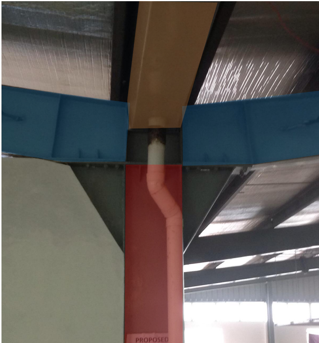
Column-rafter connection at valley
