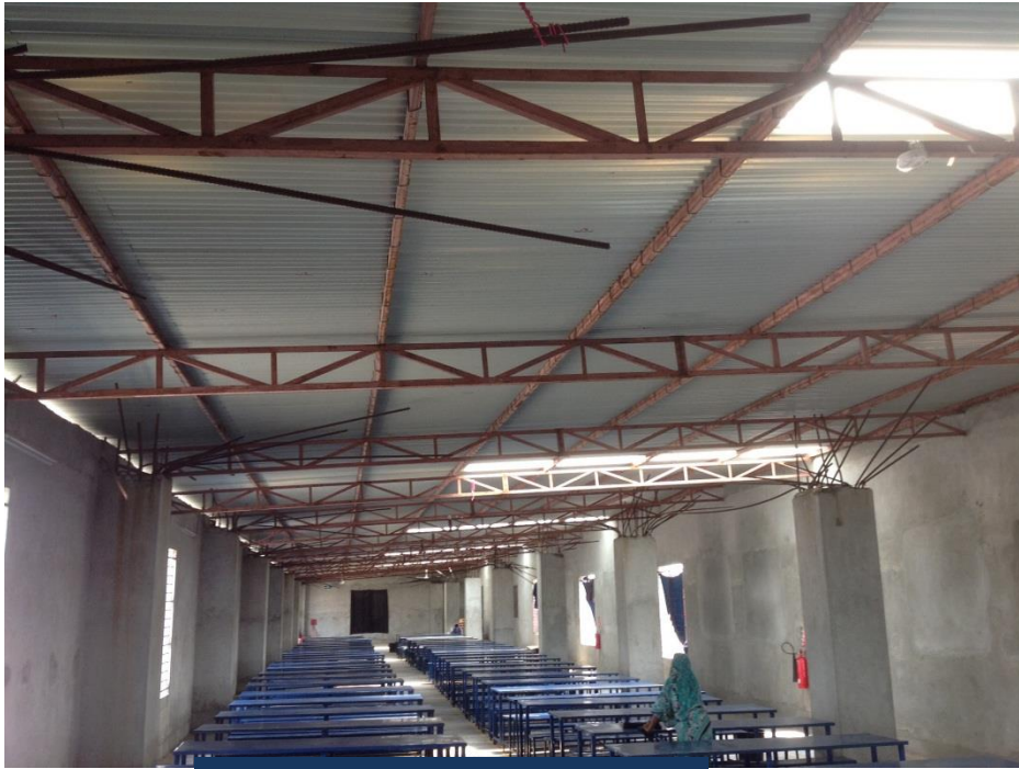
Dining area at roof level
