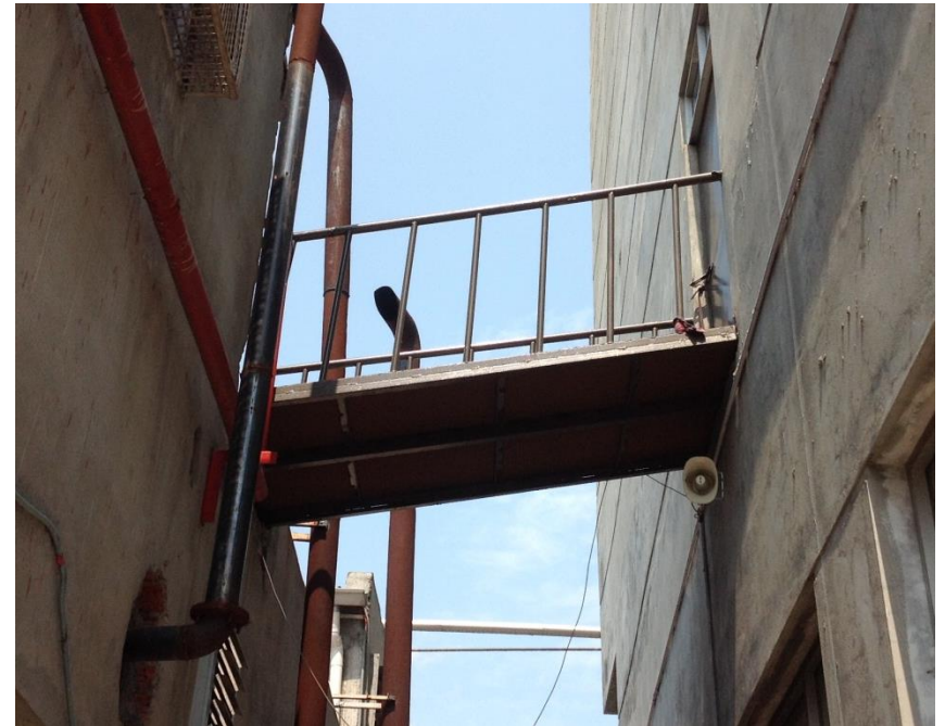
Link-bridge to rear of building
