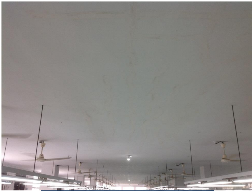
Repairs to soffit of 4 th floor slab
