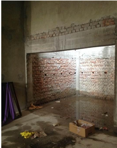
Lift shaft opening
