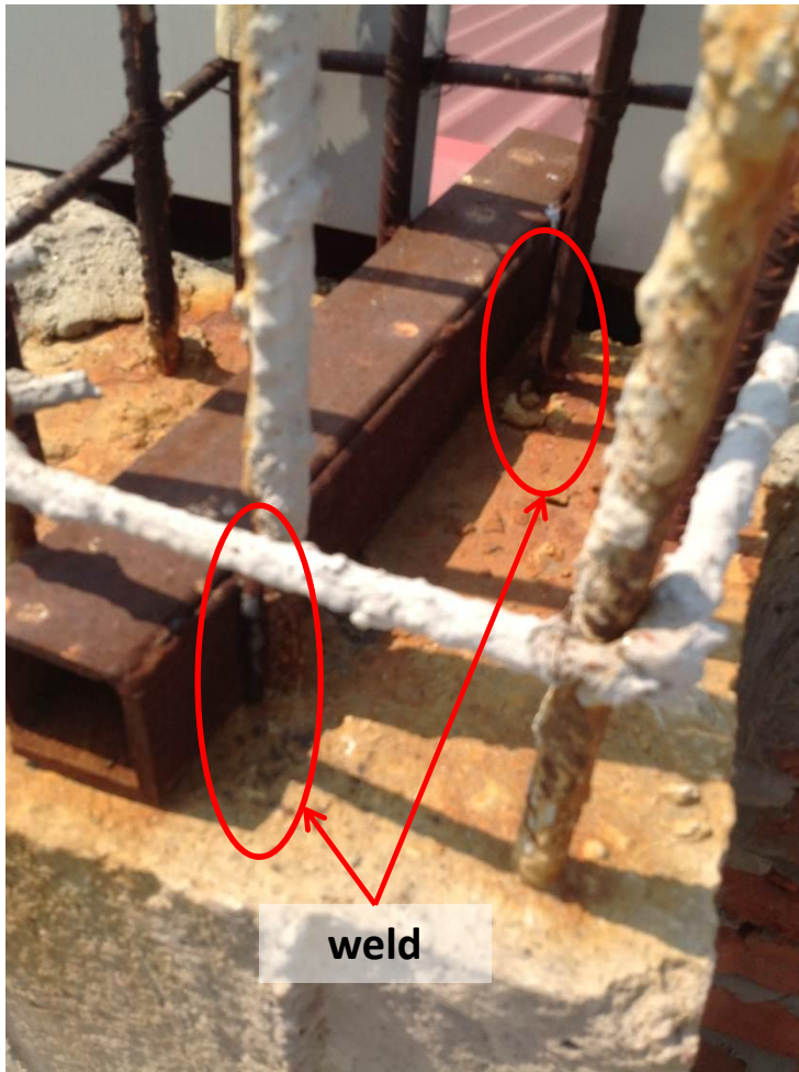
Canopy bracket welded to rebar
