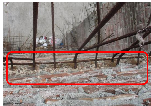
Brick aggregate observed
