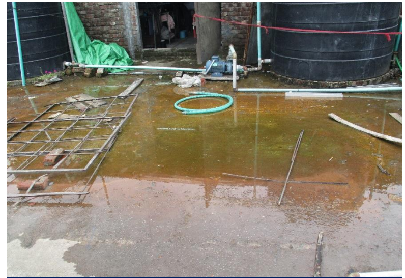
Water ponding at roof
