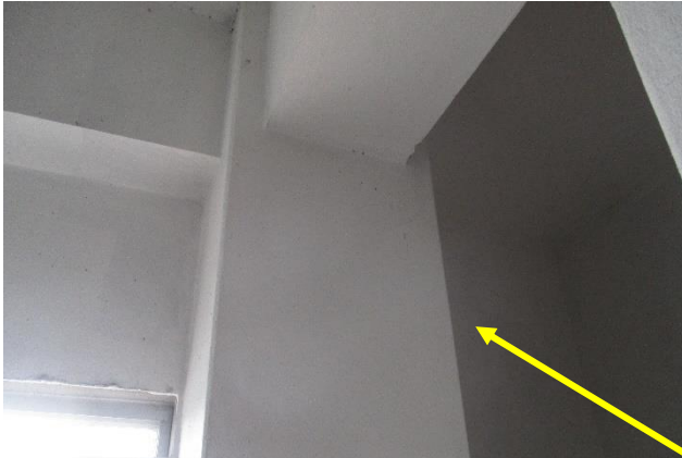
Cantilever without beam
