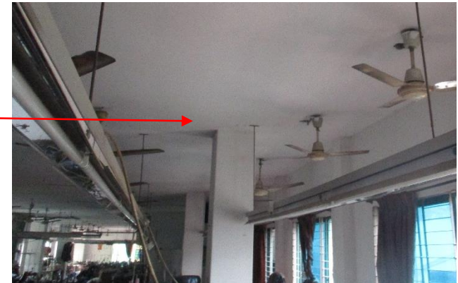
Flat slab up to 2 nd floor
