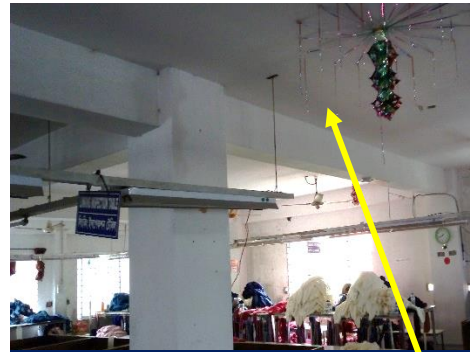
Floor beam at part-B
