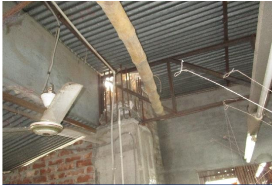
Roof shed with truss
