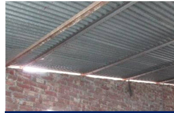
Stair core roof
