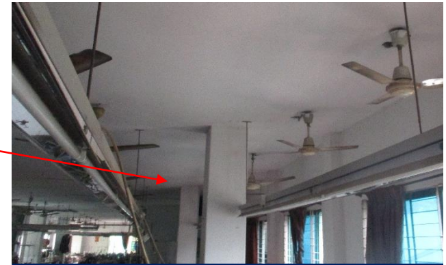
Flat slab up to 2 nd floor
