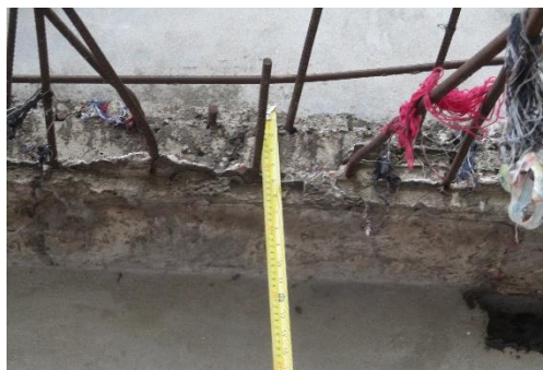
Brick aggregate observed
