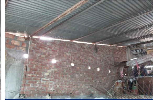
Stair core roof
