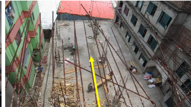
Up to 1 st floor construction at part-C
