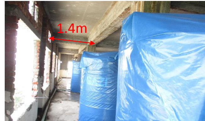
Cantilever at South
