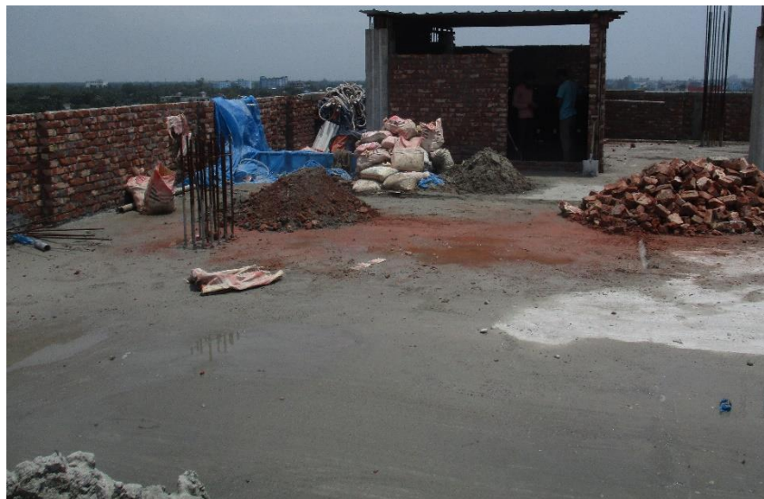
On going construction work at roof
