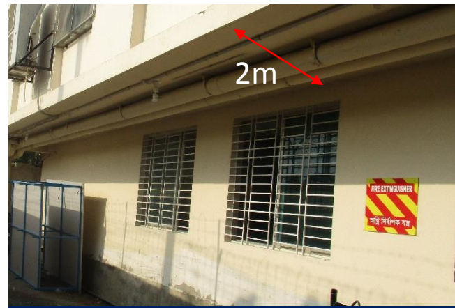
Cantilever at west
