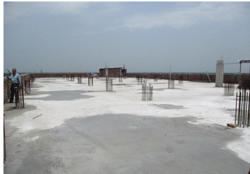
Newly constructed roof slab
