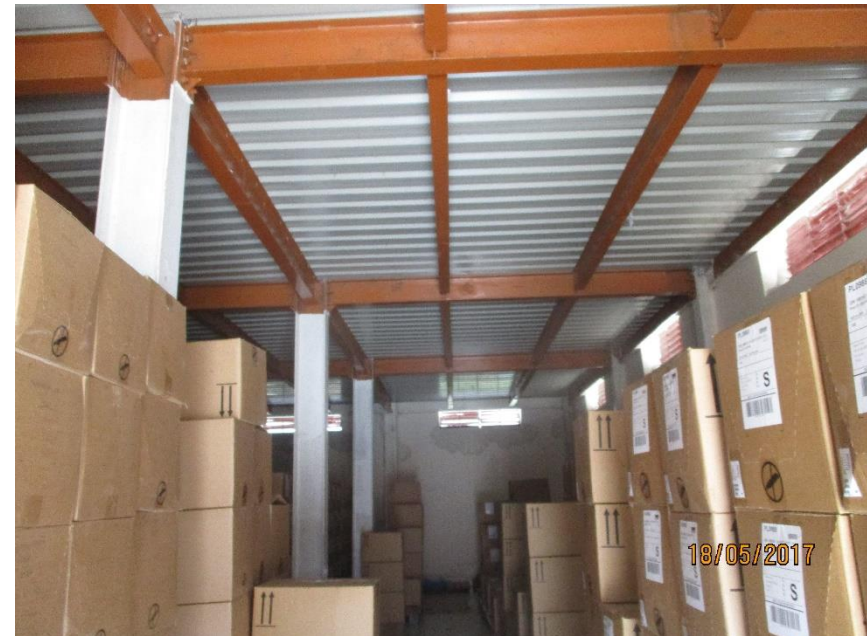
Finish good storage building
