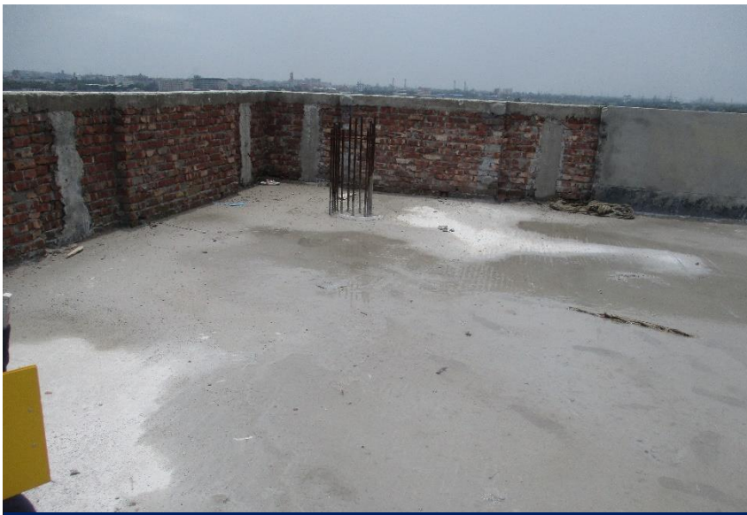
Signage of water applied for curing
