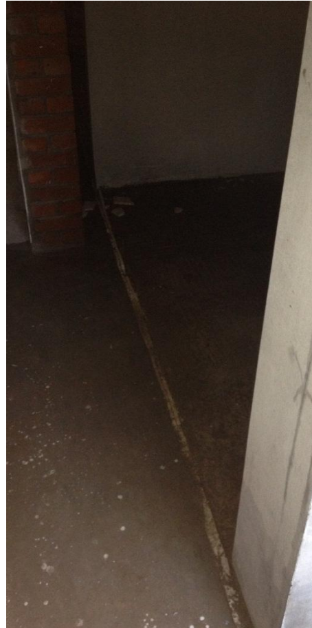
Existing movement joint between Building No.1 and 3
