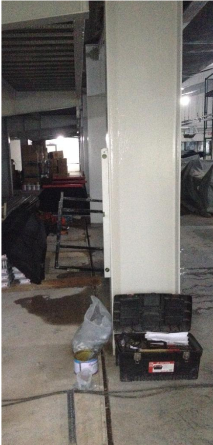
Existing movement joint between Building No.1 and 2
