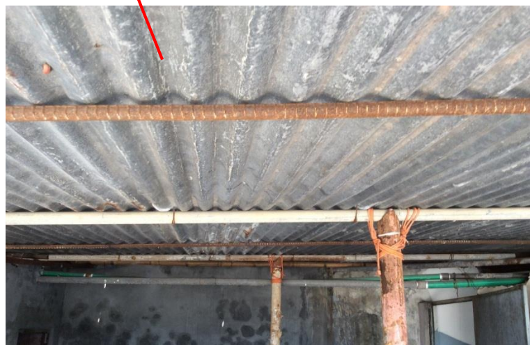
Steel roof supported by bamboo and rebar
