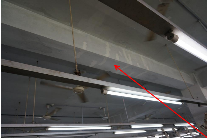
Crack repairs on beams supporting roof slab
