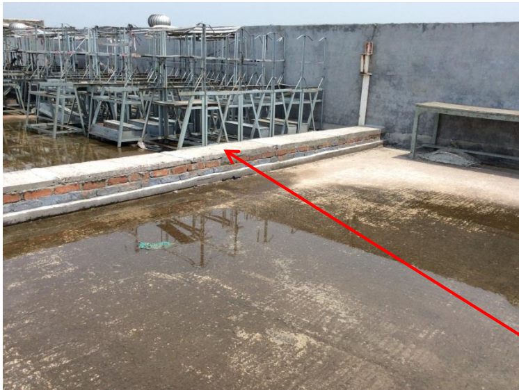
Movement joint on roof
