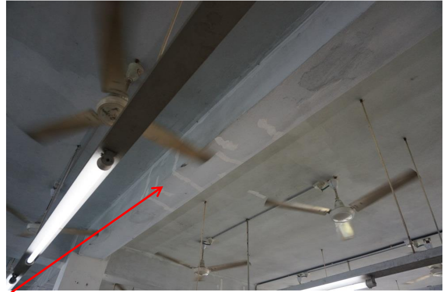
Crack repairs on beams supporting roof slab
