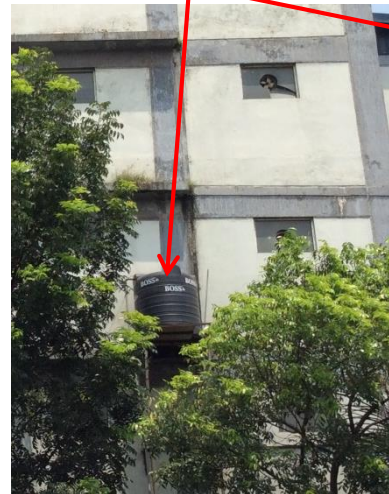
Steelwork supporting water tank at east façade.
