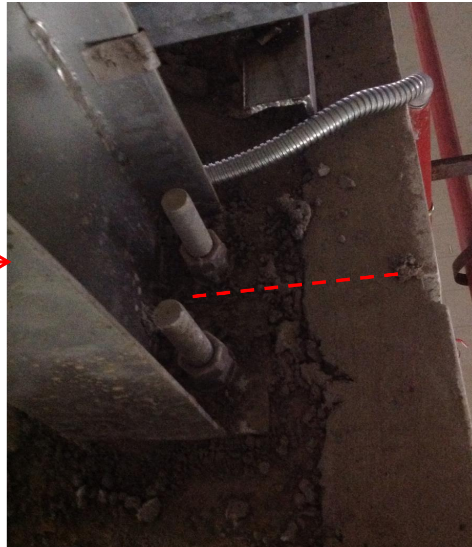
Baseplate anchored both sides of movement joint
