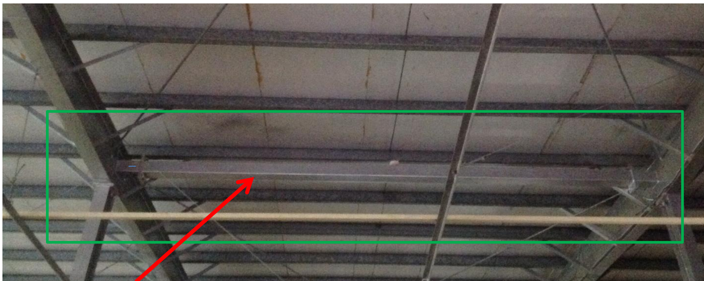
Compression strut in roof bracing
