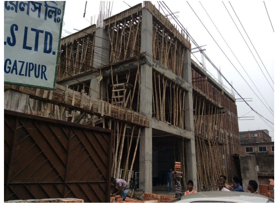
Peak Apparels was under construction at the time of survey. The RC frame had been constructed up to 4 th floor slab.
