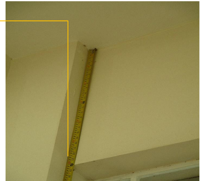
Several beam sizes doesn't match with provided drawings.
