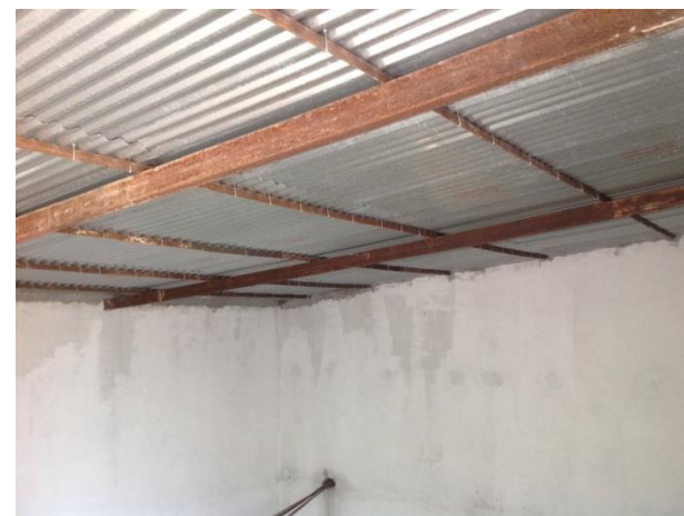
Roof of the staircase in the main building
