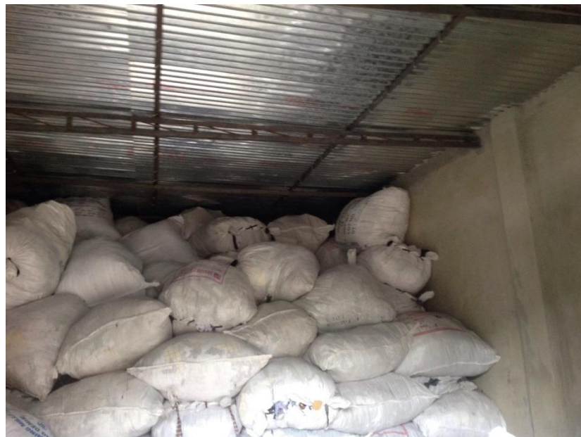
Storage shed roof structure
