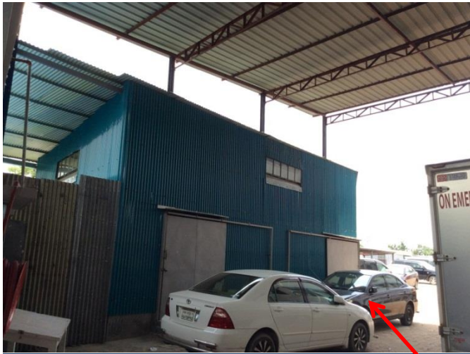
Steel Roof spanning between the Main Building and Childcare Building
