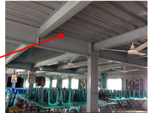
Steel roof of Main Building
