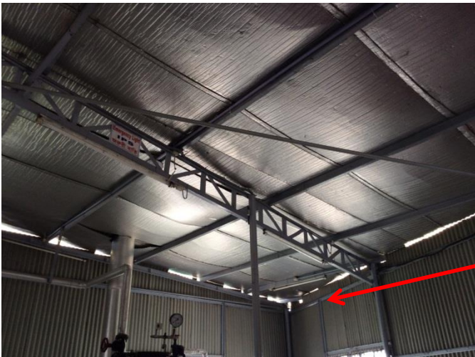
Steel roof of Utility Building
