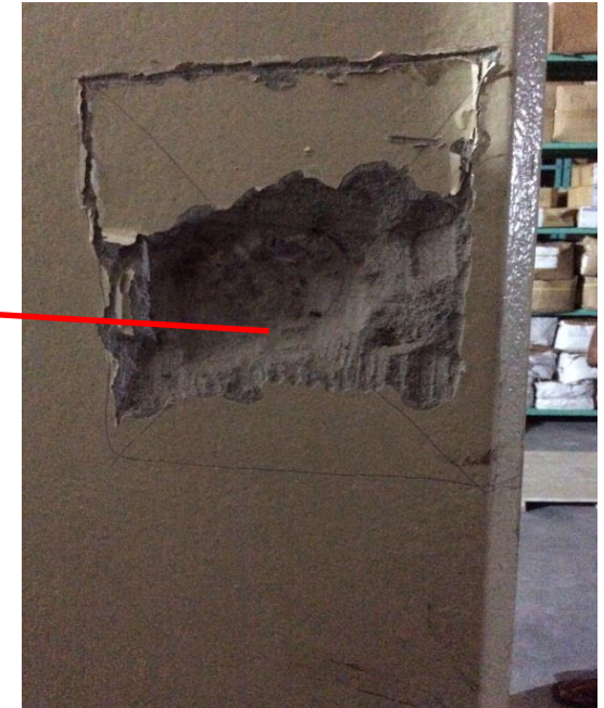
Column Test - Stone Aggregate
