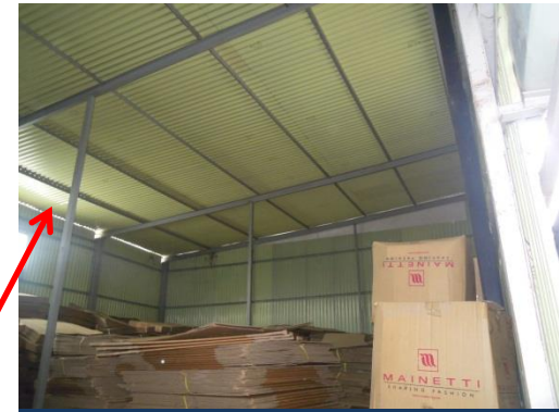
Light steel roof to Storage Building
