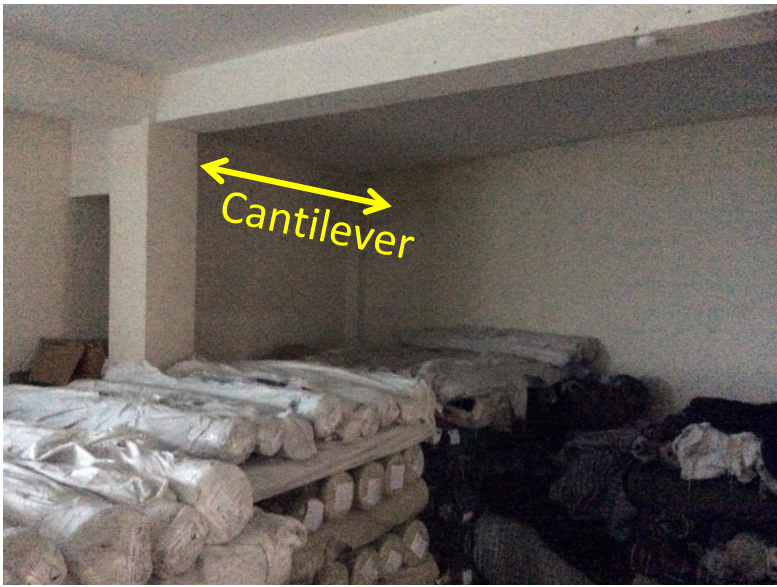
Large storage loading on Cantilever slab.
