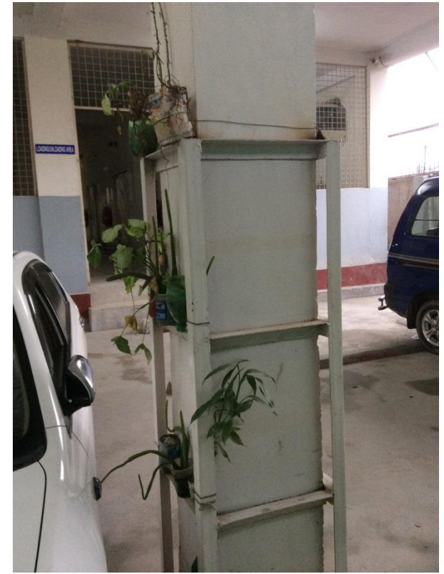
Current column protection
