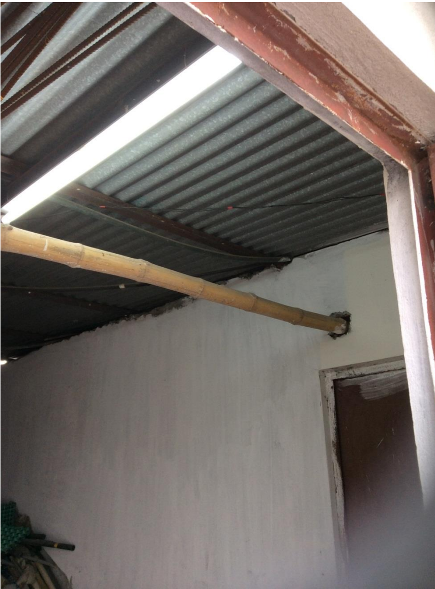
Non-Engineered Steel Roofs to Stair Cores.
