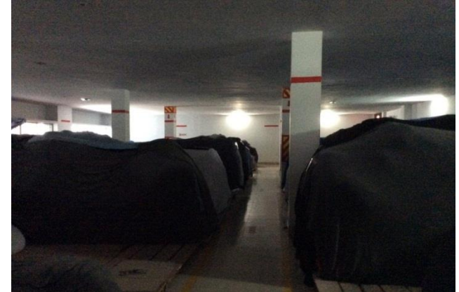
5 th Floor Material storage – Load height limits indicated on columns are not based on calculations
