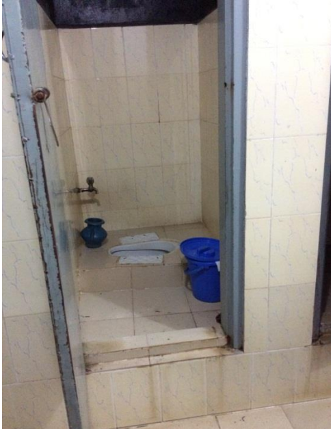
Toilet build-up on suspended slabs
