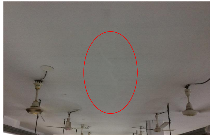
Repairs to soffit of 3 rd floor slab
