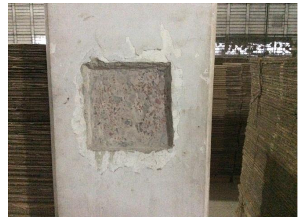
Tested ground floor column – Brick aggregate confirmed
