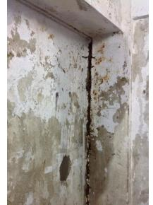
Movement joint exist at centre of structure, spanning in the North to South direction.
