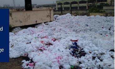
**First Floor** Uncontrolled / unrestricted loading observed on first floor.
