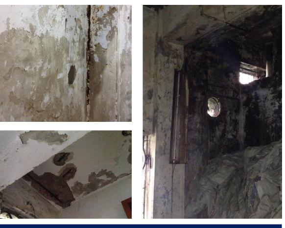
Extensive water ingress at roof level causing deterioration of structure.Water ingress causing spalling to beams, slabs and columns throughout structure, particularly on 1st Floor.
