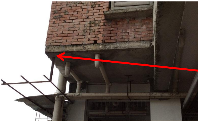
North Elevation Slab Cantilever
