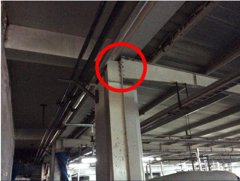
Laundry Room LW Steel Roof Frame
