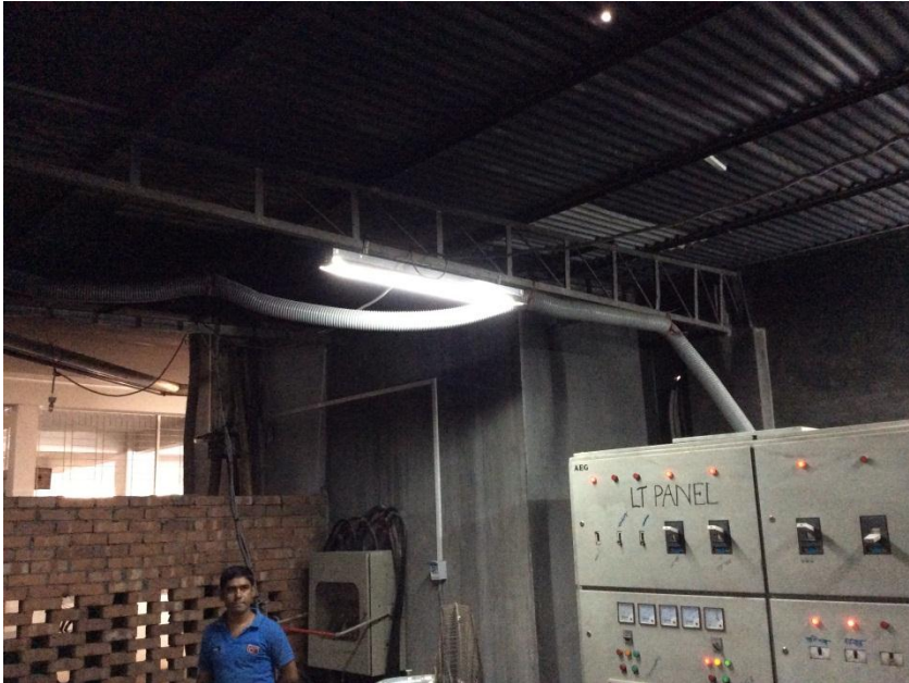
Transformer and Switch Room LW Roof Structure
