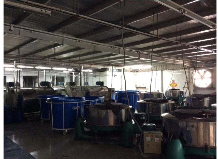
Laundry Room LW Steel Roof Frame
