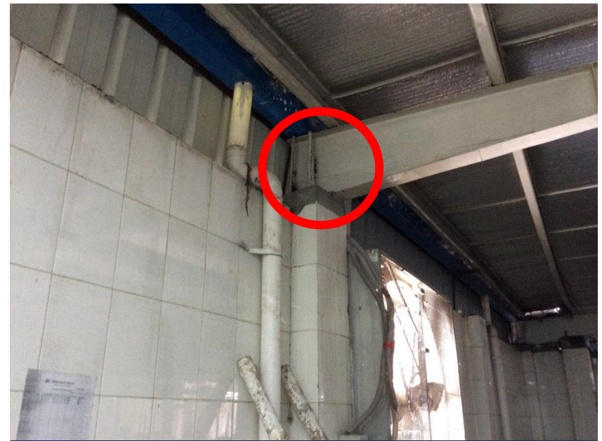
Laundry Room LW Steel Roof Frame
