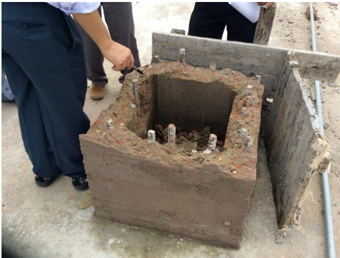
Column Reinforcement at Roof Level
