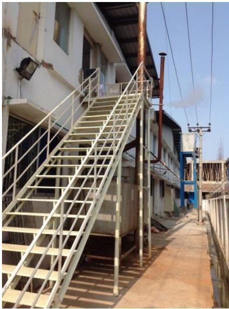
Fire escape stairs outside the building (5 no.): poor structural details and weld quality
