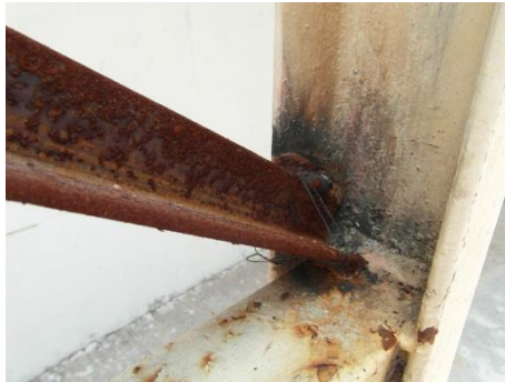
Fire escape stairs outside the building (5 no.): poor structural details and weld quality
