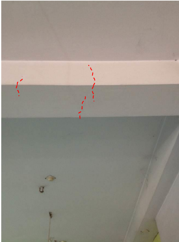
Beam cracking
