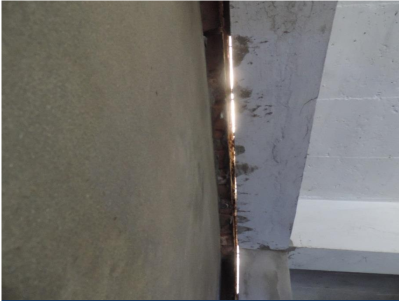
Soffit of 1 st floor beam
