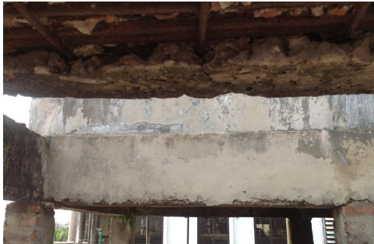
Water tank supporting beam
