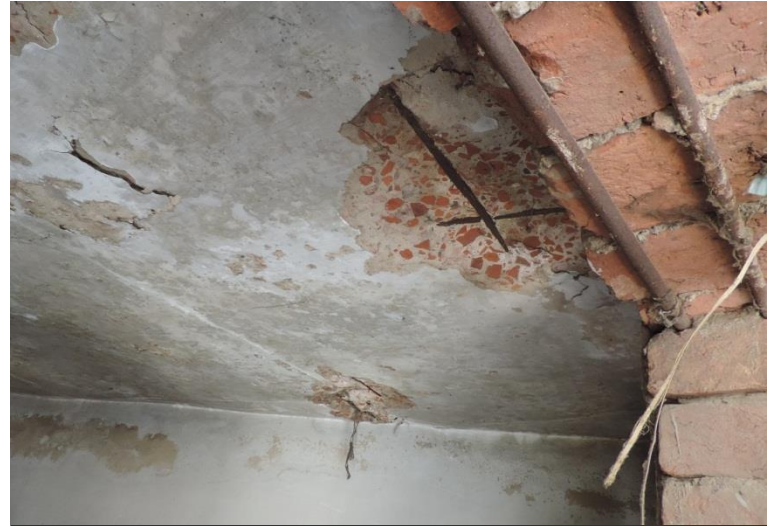
Soffit of boiler house roof slab
