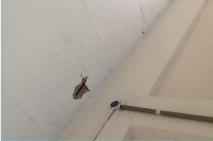
Soffit of cantilever slab
