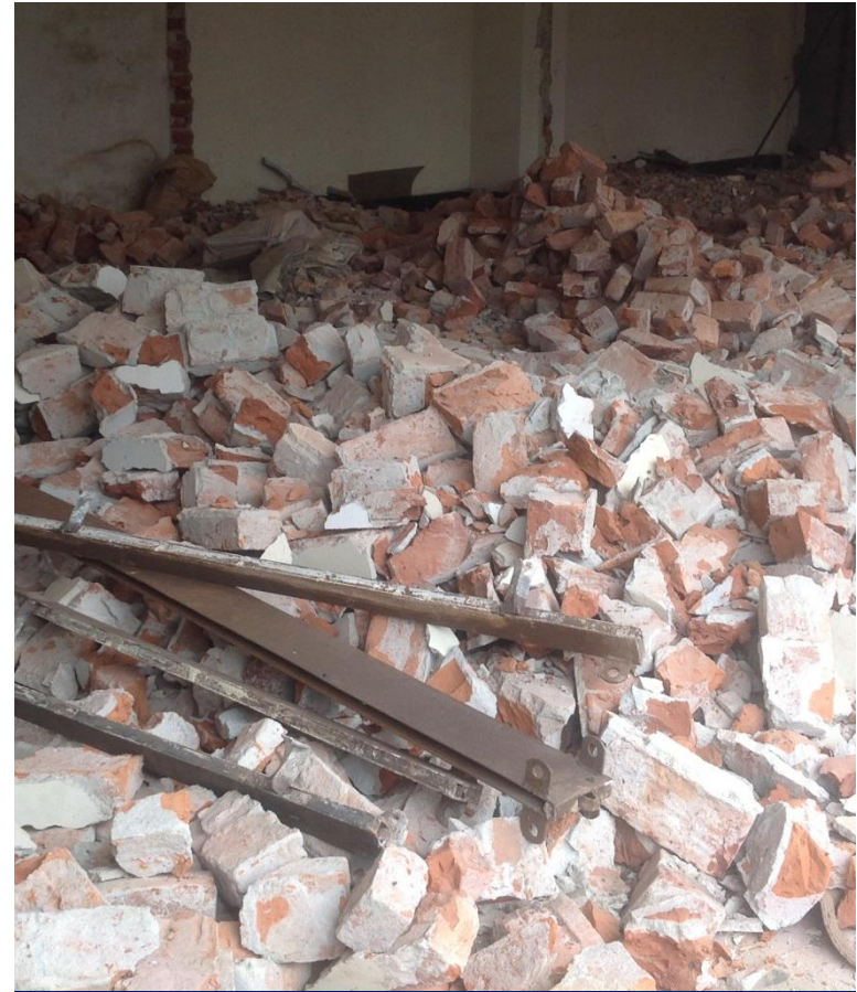
Rubble from brick wall demolition
