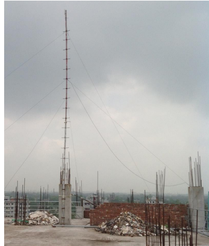
Mast and unreinforced masonry wall
