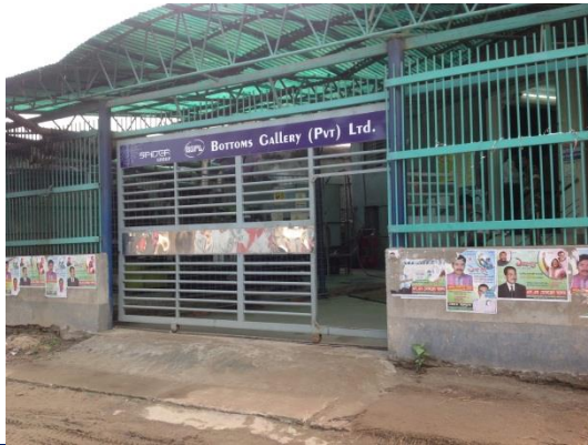
Steel roof to generator
