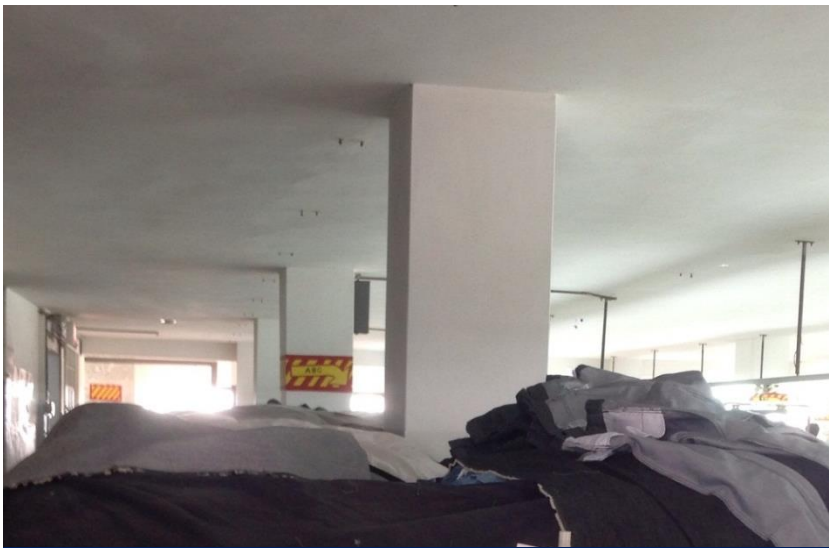
Critical Internal Column at Level 5
