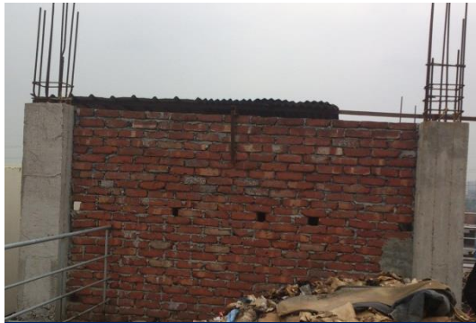
Unreinforced masonry wall
