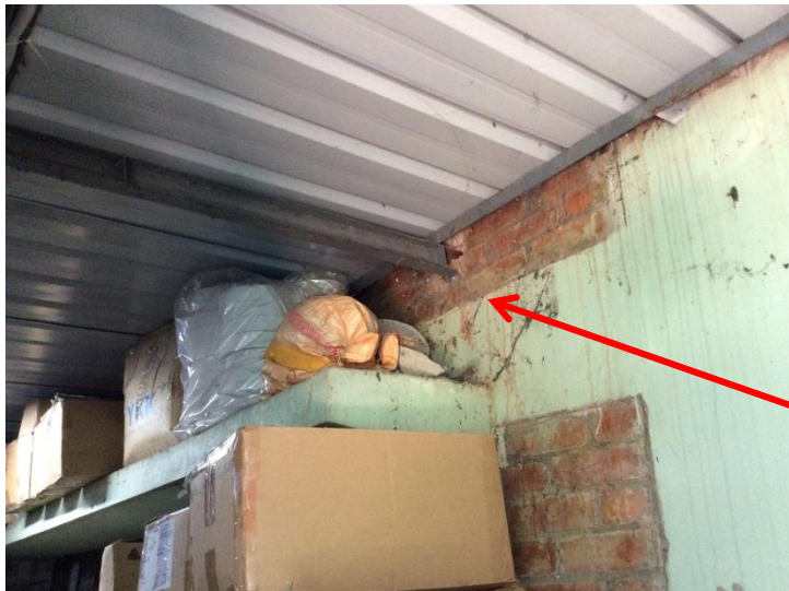
Canteen: missing bracing
