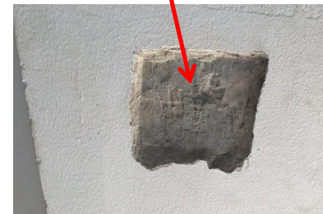
Tested Ground Floor Column – Stone Chips
