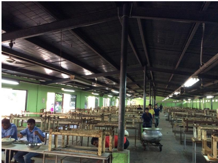
Canteen: missing bracing
