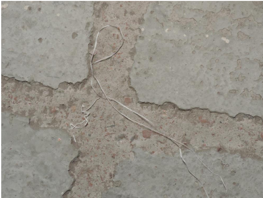
Brick aggregate in slab 1 st floor
