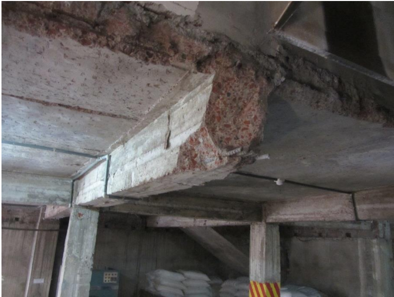
6 Columns removed leaving beams cantilevering
