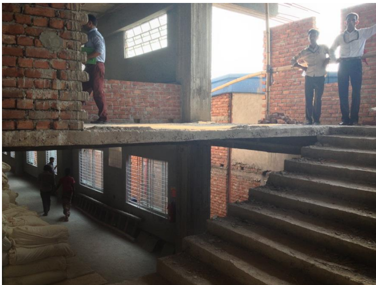
Missing beams around stair
