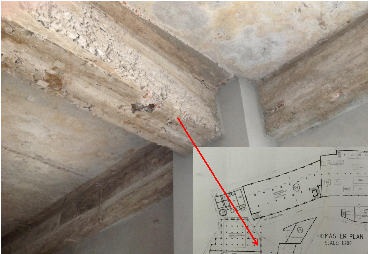
Building 5 – Very poorly compacted beam
