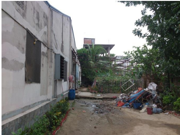
Open lattice to South Elevation – Shed 1
