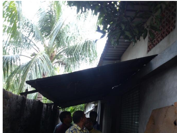
Lean-to cover to the West Elevation – Shed 1
