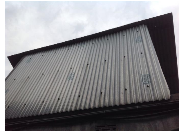
Roof extension over generator
